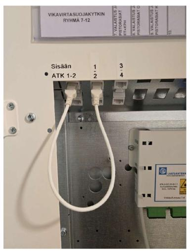
In the picture, the computer socket is connected via a data cable (RJ45) to apartment socket number 1. if needed, you can switch the connection to sockets 2, 3, or 4.
